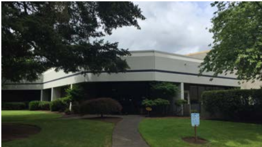
API Headquarters - Office Building
