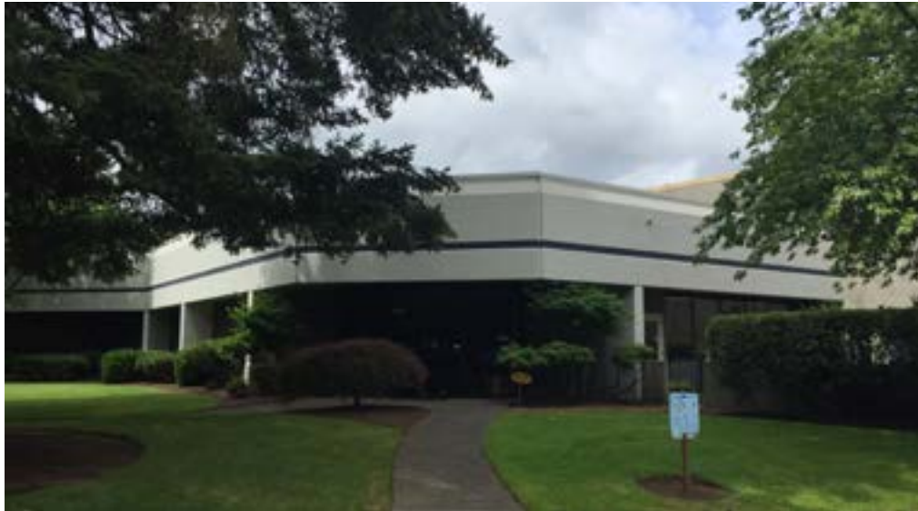
API Headquarters - Office Building
