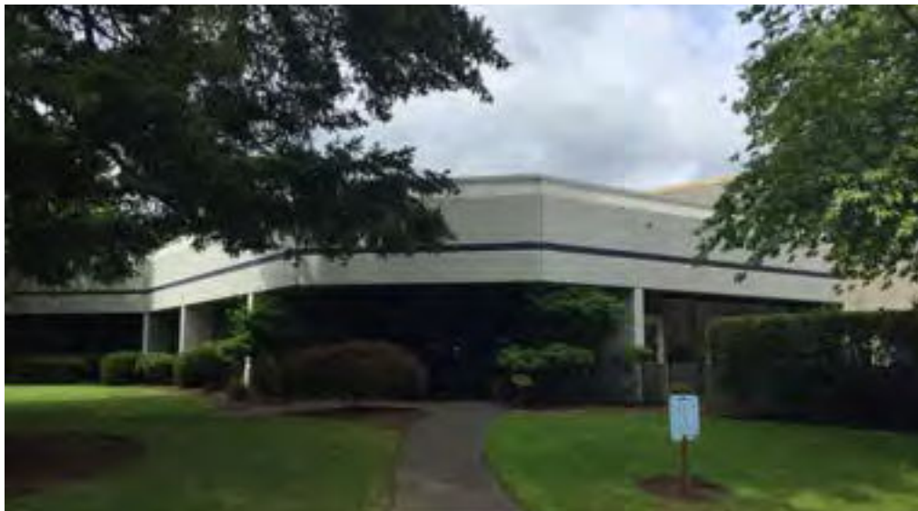
API Headquarters - Office Building
