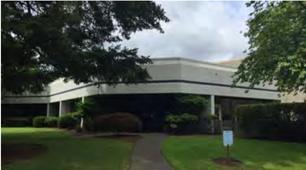
API Headquarters - Office Building
