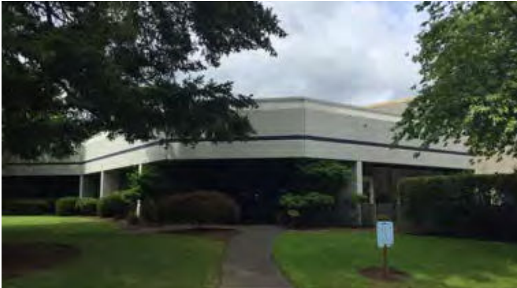
API Headquarters - Office Building
