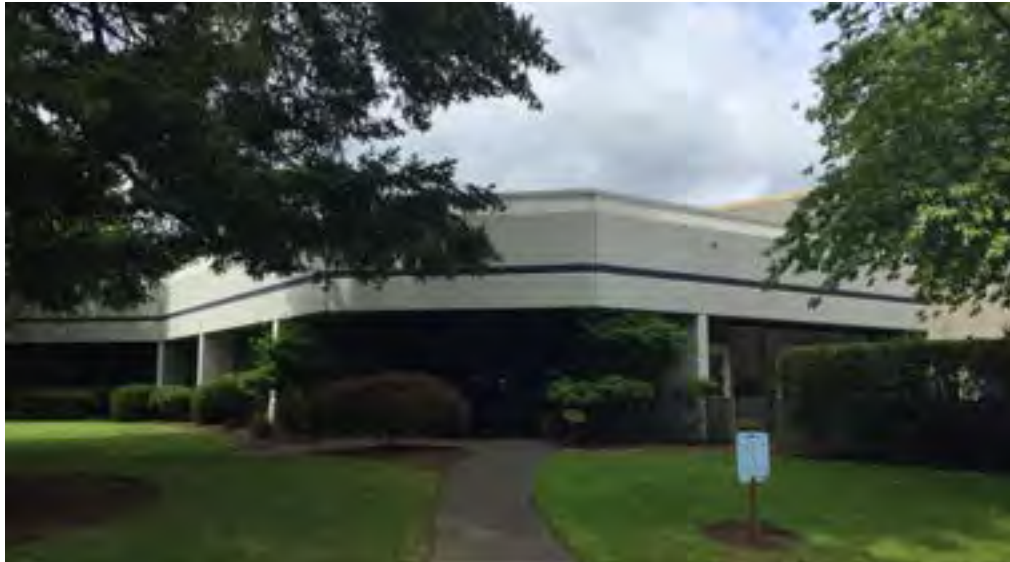
API Headquarters - Office Building
