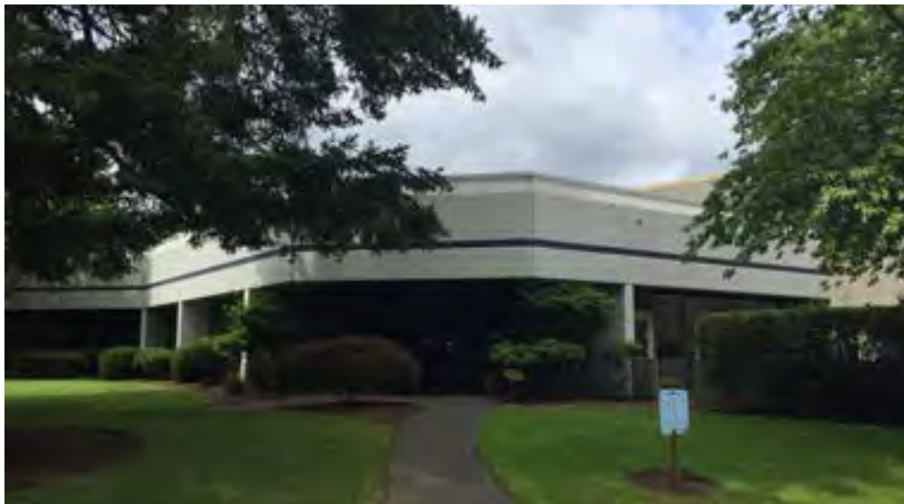
API Headquarters - Office Building
